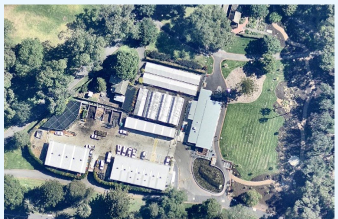
↑ After: 5,000m 2 depot area, new 4,000m 2 open space, a new visitor centre and a 5ML underground water storage tank
